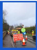
Operate units in line of sight of full set up at all times. Press any button to bring all to STOP. The designated button will bring allocated sign to GO position.
